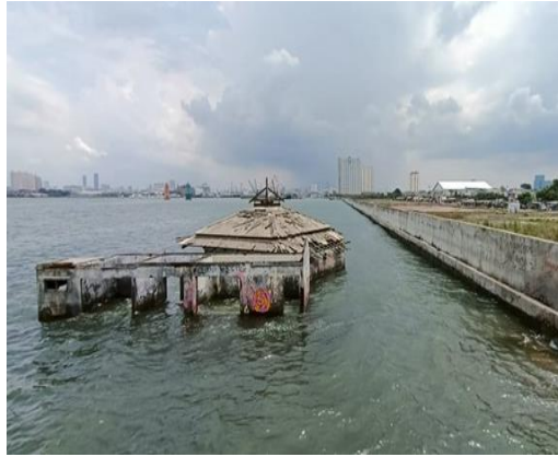
Figure 7. Sinking area at Muara Baru (source: google, 2022)
